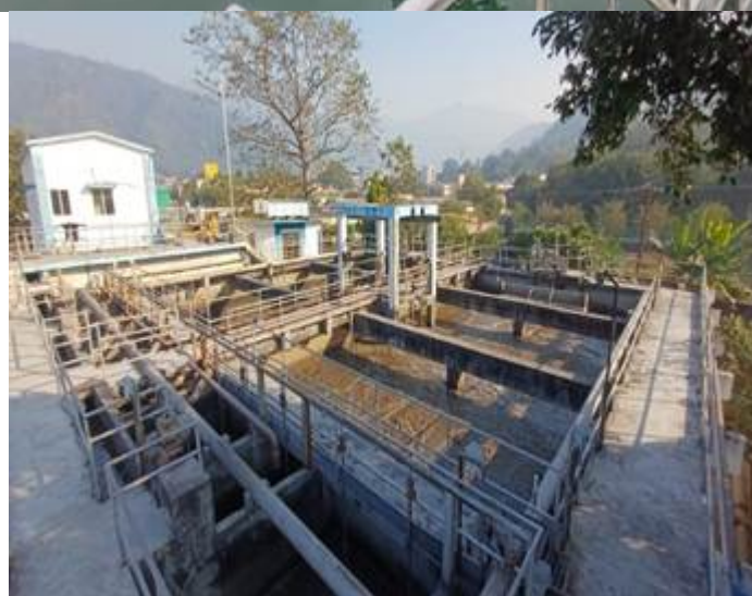
8 MLD STP at Muni ki Reti
