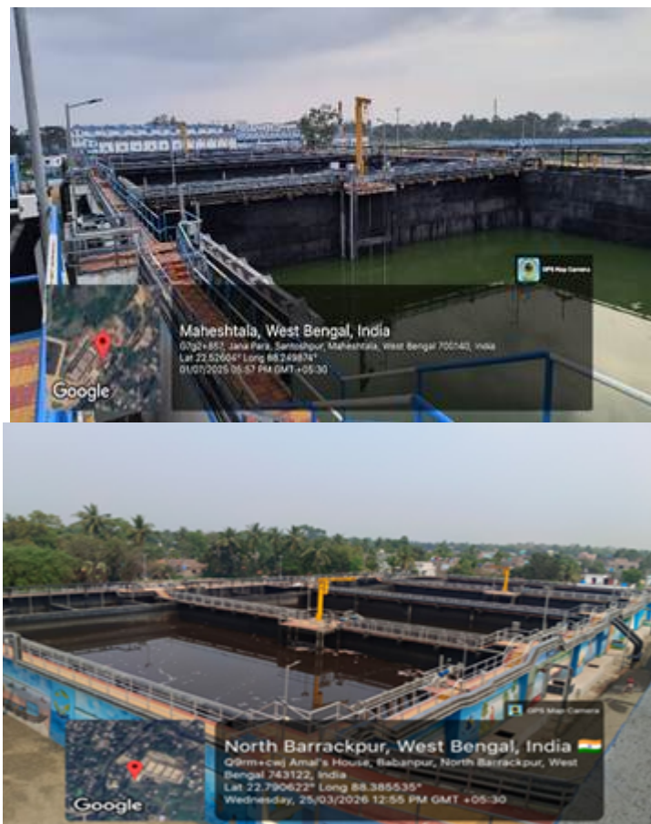
35 MLD STP at Maheshtala
